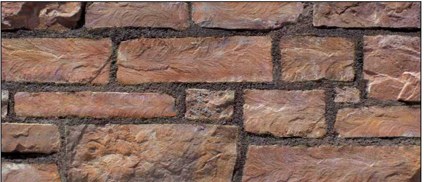
½" Deep Raked Grout Joint
